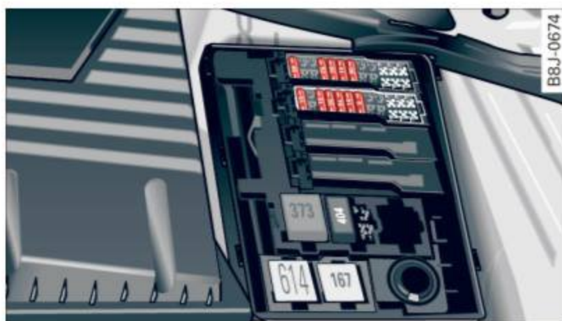
Fig. 167 Illustration of fuse holder on left side of engine compartment: fuses (without fuse cover)
